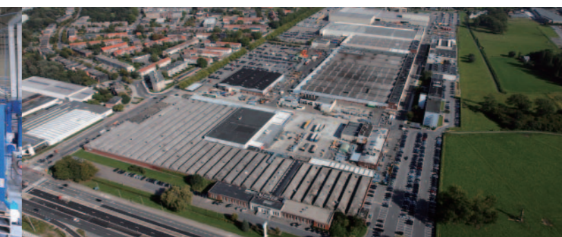
Oil and water injected screw compressors plant: Belgium
